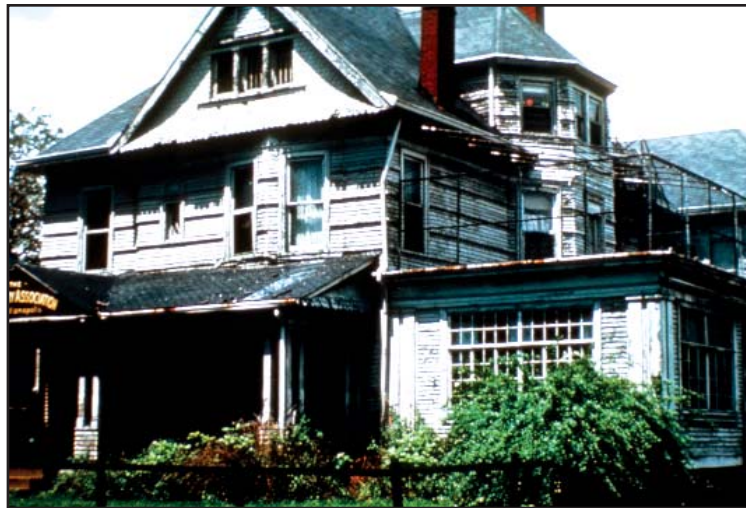
◀ One of the many "before" photos of the former Day Nursery Association facility which the Smalls began renovating in 1971. Note the addition at the right (with railing on top), which was removed. It was not original to the house.
