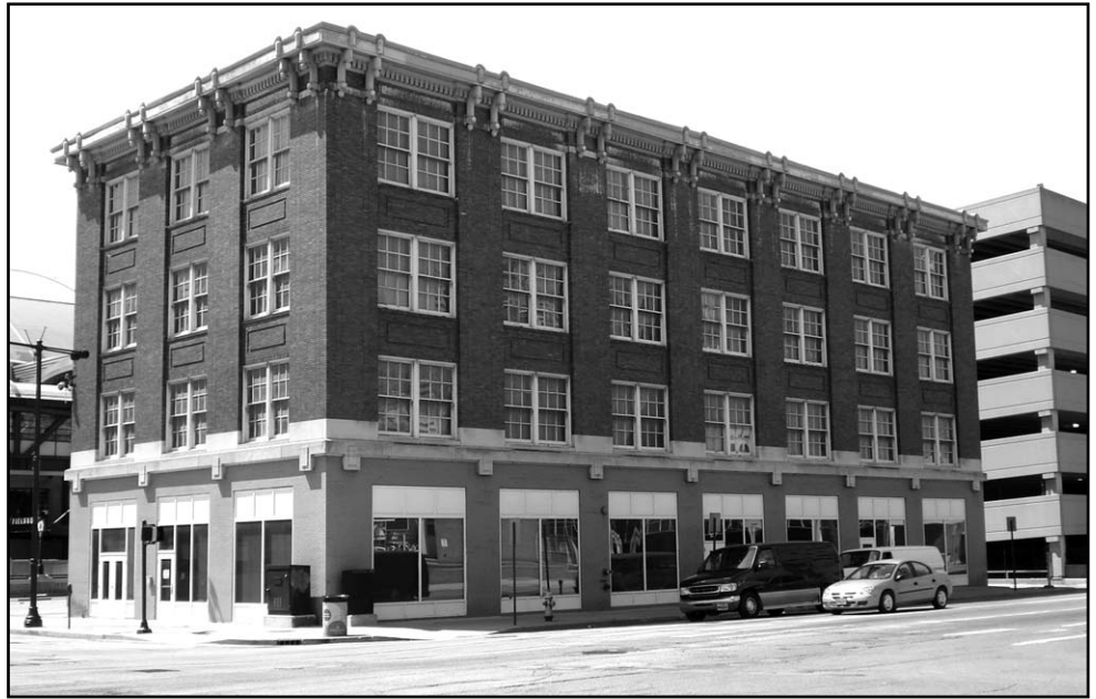
▲ Canned vegetables were produced under the Ko-We-Ba brand in this Delaware Street building located just north of Conseco Fieldhouse.
