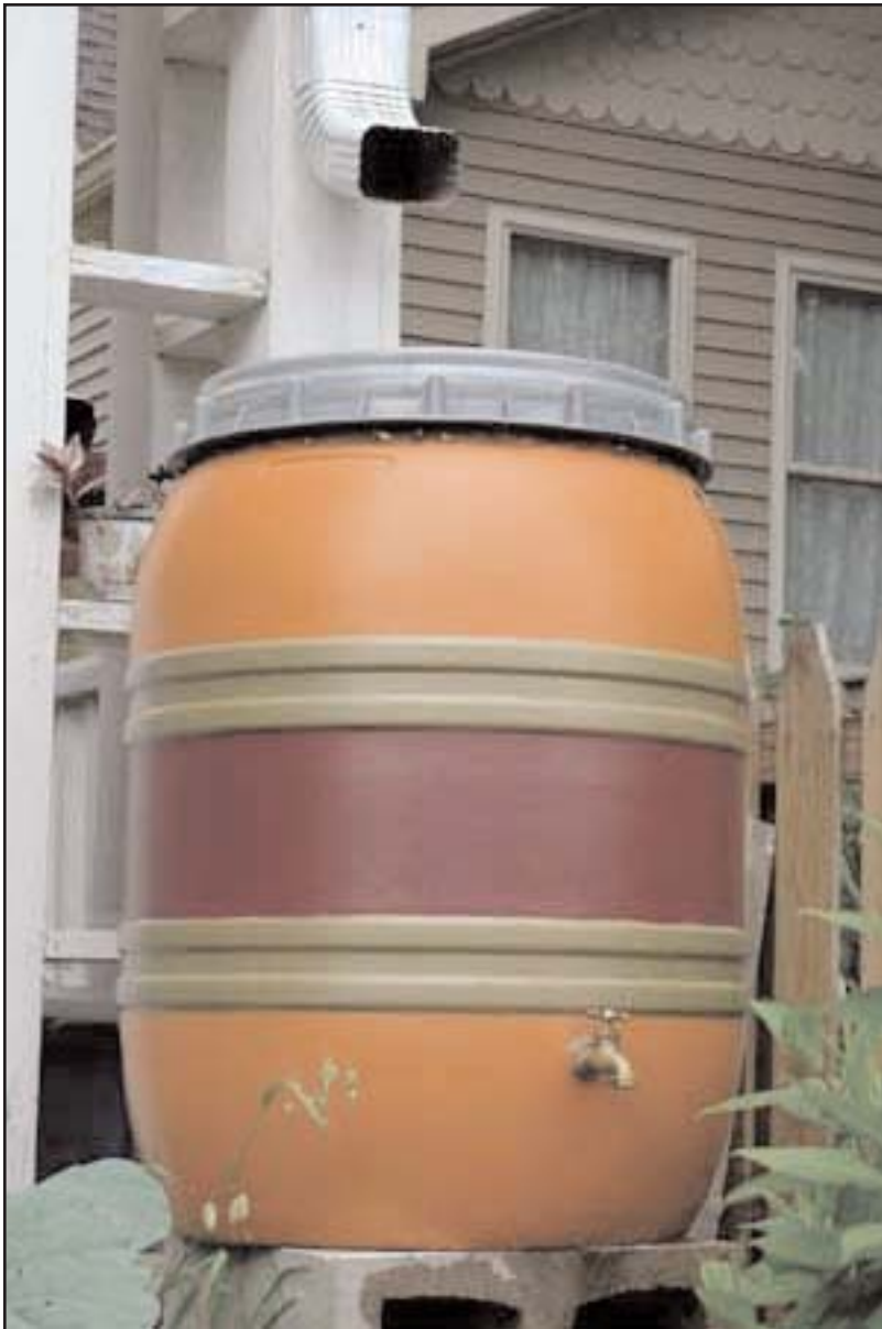
▲ The finished product: A rain barrel which collects water from downspouts, and features a tap which the homeowner can use to recycle the water.
